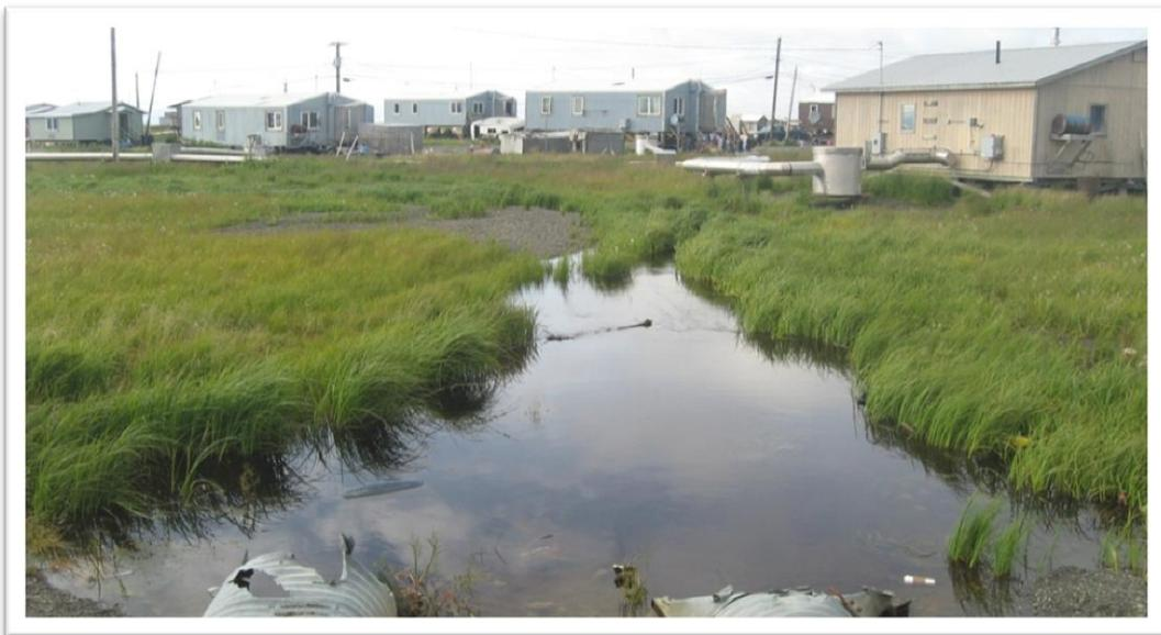
Figure 4. Downstream side of two 24" culverts under Old Quinhagak Airport Road (Qunirtuuq Drive). Note the large sediment deposits carried into the wetlands below the road.
