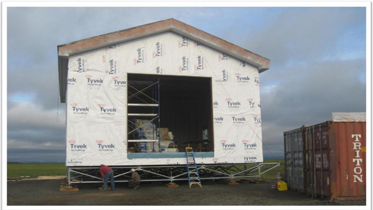
Figure 24. Jeff Hoffman inspecting Triodetic foundation system on new Community Service Center being built for Coastal Villages Seafoods (CVS).
