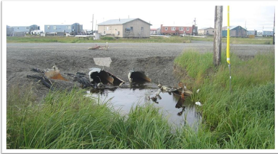
Figure 3. View is to the north at two 24" culverts under Old Quinhagak Airport Road (Qunirtuuq Drive) near intersection with Agalik Avenue. Road has been over topped and washed out.
