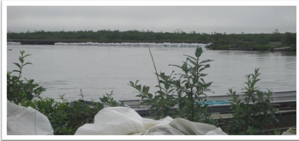
Figure 1. Super sacks foreground, and in the distance, along Kanektok River shoreline adjacent to the old airport runway placed in an attempt to curb erosion.
