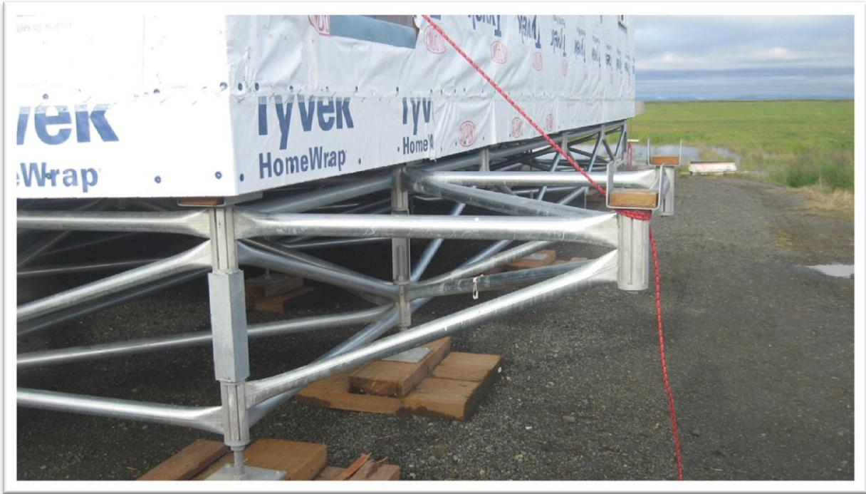
Figure 25. Close-up of new Triodetic foundation system under Community Service Center building.
