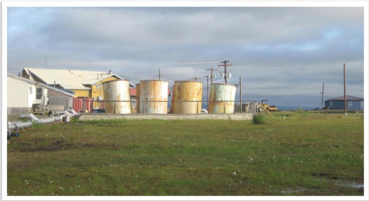
Figure 18. AVEC tank farm. Note: the tilt of the tanks.
